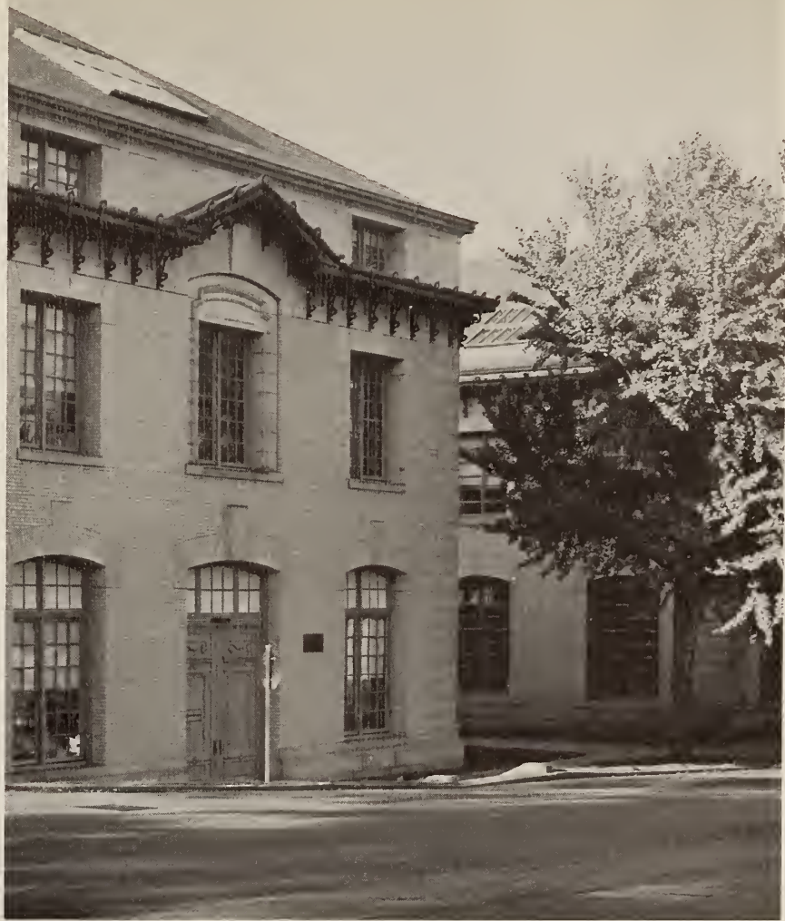
Wires, pipes and Black Magic.
